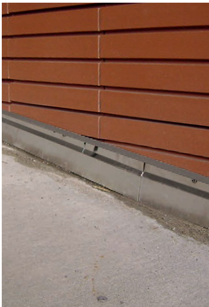
Lower finish with aluminium sheet
