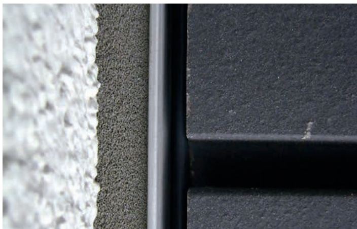
Inside corner Argeton/plaster
