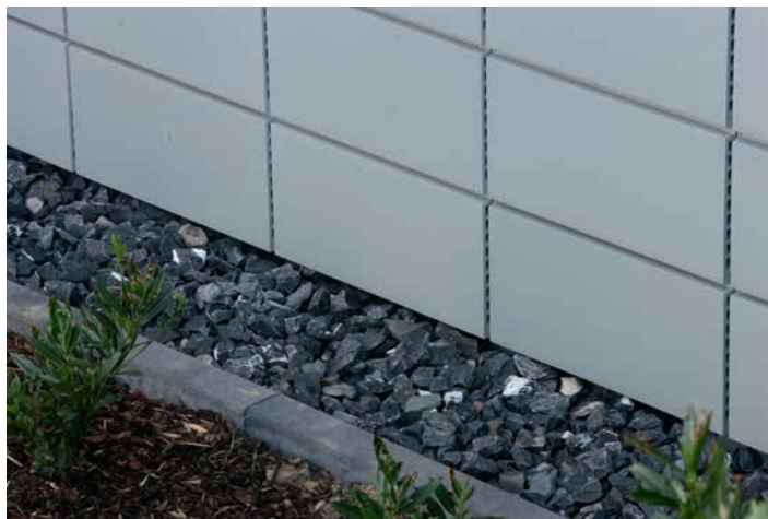
Lower finish with aluminium sheet
