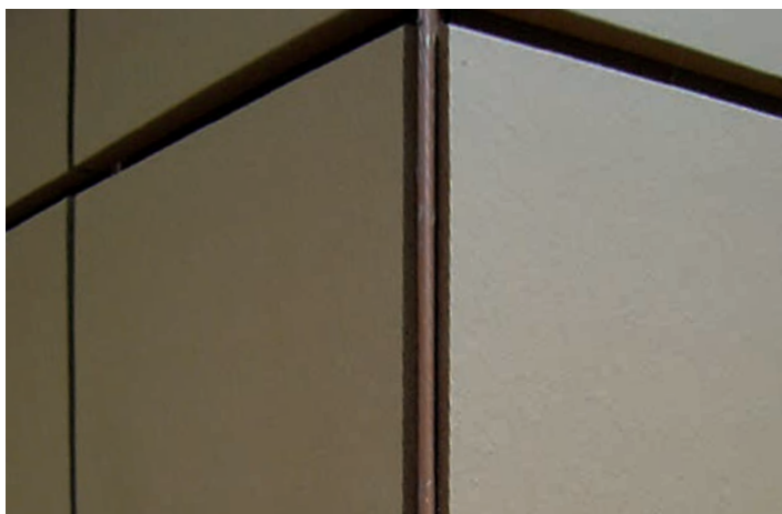
Inside corner Argeton/plaster
